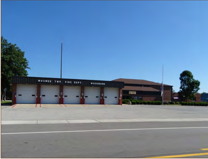
City of Woodburn City Hall and Fire & EMS Station
