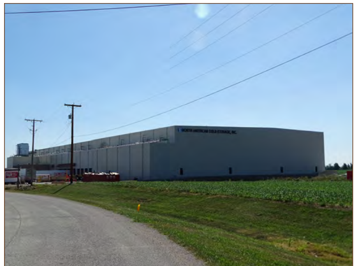
North American Cold Storage, Inc. - Woodburn Industrial Park
