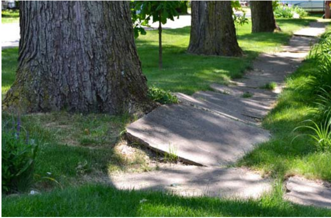
Grade F – Not present, broken, and/or impassable.
